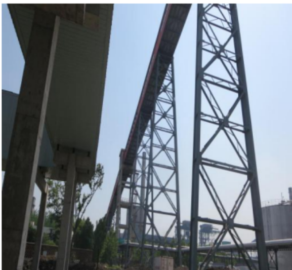
封闭式煤转运通廊
